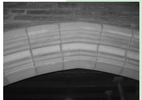
Repairs to the entrance arch at the Phi were made this year by pro stonemasons. The completed arch, seen above, should last another century.
