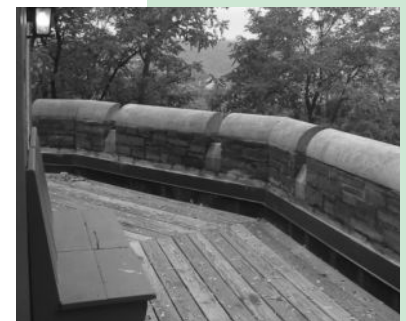
Phi Lodge Roof Deck
