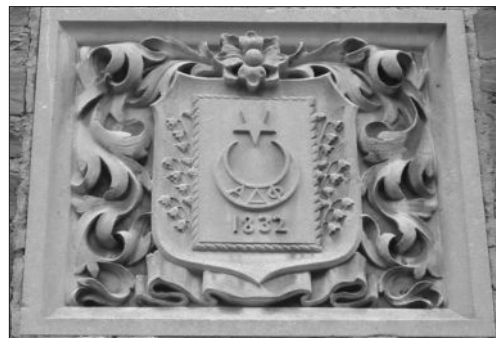
Exterior stonework AΔΦ crest
