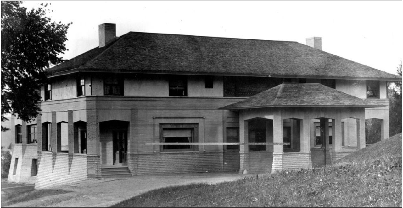
Alpha Delta Phi photographed after the new lodge was completed.
